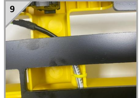
Secure the extension cables to the step using the 12 small cable ties. (PRO-PARK-AM10Y Shown)
